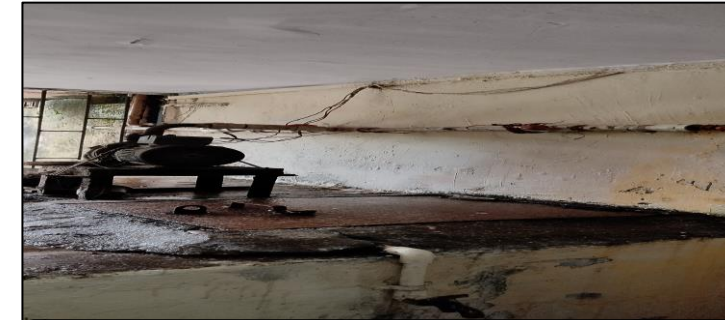
Water Tank - Ground
